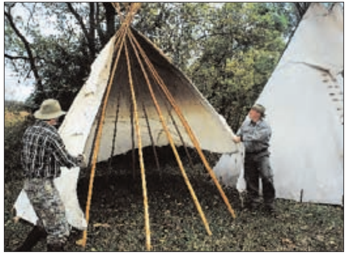
Ramshaw sewed his tipi cover from canvas tarps in a semi-circular pattern obtained from a book.
