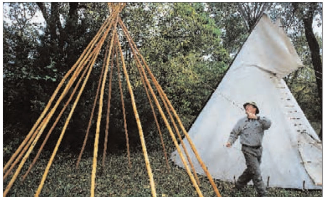
There is an art to setting tipi poles. Beginning with a simple tripod twisted with rope at the top, remaining poles are added and wrapped together.
